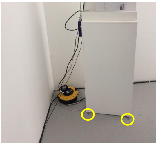
Circled in yellow in the picture are brackets that have been used to secure the plinth to the floor.
